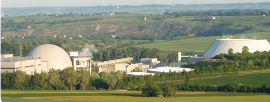
Example of a circular hybrid cooling tower (far right) at Neckarwestheim nuclear power station in Germany. Similar cooling towers could be used for the Oldbury site. Picture by Thomas Springer
